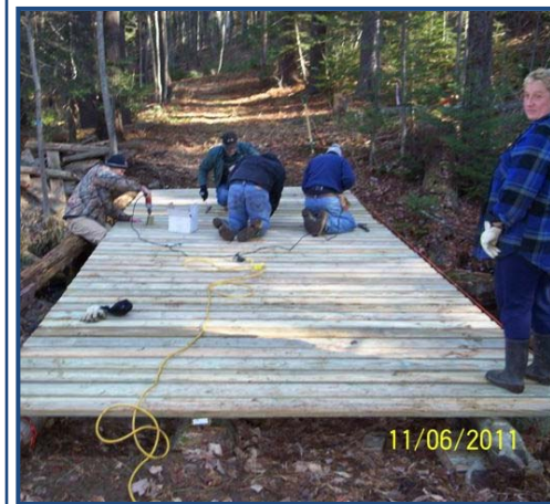
Building a new bridge on ITS 87 just before the Rt 202 crossing
